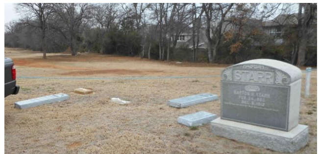
We dug out and discarded the two old bases. Only a little more digging was needed to make footing holes for the new rocks.
